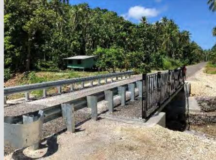
The NiuBridge modular bridge system is a light weight system for all spans up to 24m. NiuBridge is suitable for installation on a variety of existing substructures, including timber, heritage masonry, steel and concrete. NiuBridge is also ideally suitable for installation on precast spread footing abutment systems as well as the conventional piles and abutments.
