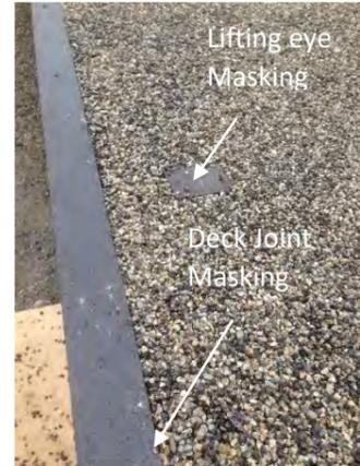
As part of the NiuBridge ECO Module design optional lifting eyes can be installed to facilitate the unloading and installation process.
